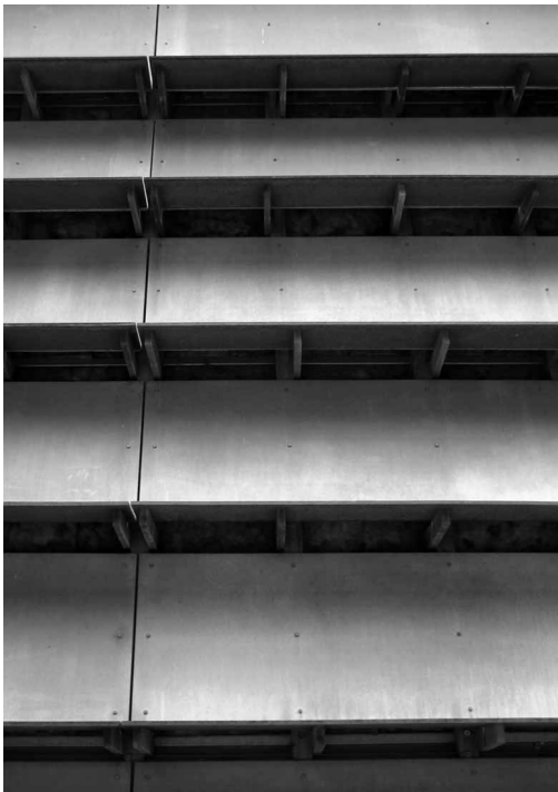
Figure 2. Stacks of planks: Ricola Warehouse, Laufen. (Photographs by James Daykin (left) and Phil Obayda (right), 2003.)
