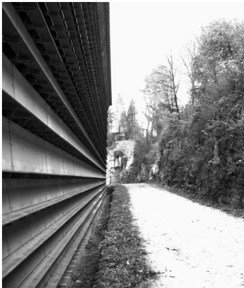
Figure 4. Between the building and the rock: Ricola Warehouse, Laufen. (Photograph by James Daykin, 2003.)
