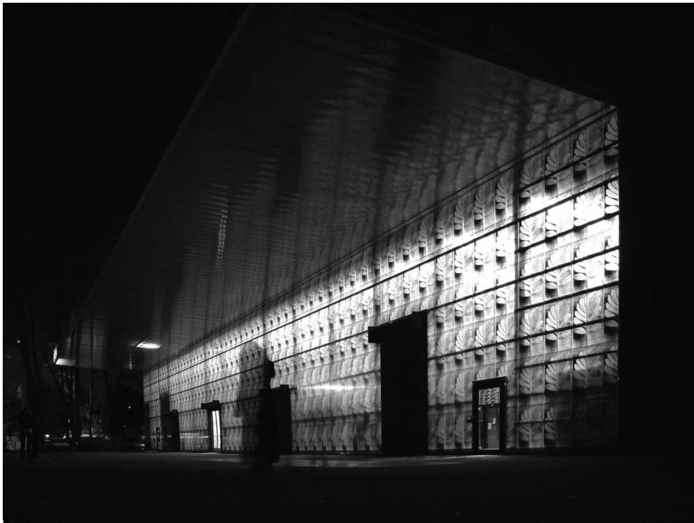
Figure 7. Night view: Ricola Packing and Distribution Building, Mulhouse-Brunstatt. (Photograph by Markus Lobmaier, 2003.)
